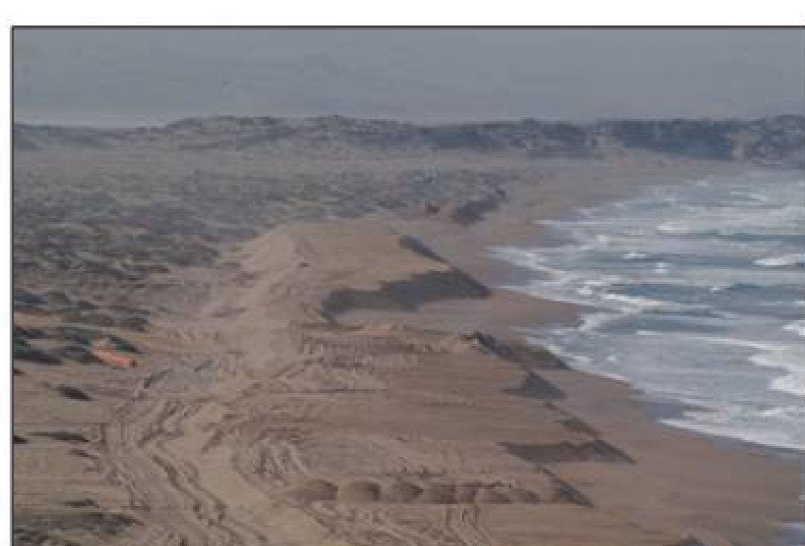
Figure 5: Pocket beach construction site at coast
